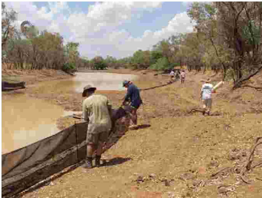
Once the fence is rolled out, the droppers (already attached) are banged into the ground.
