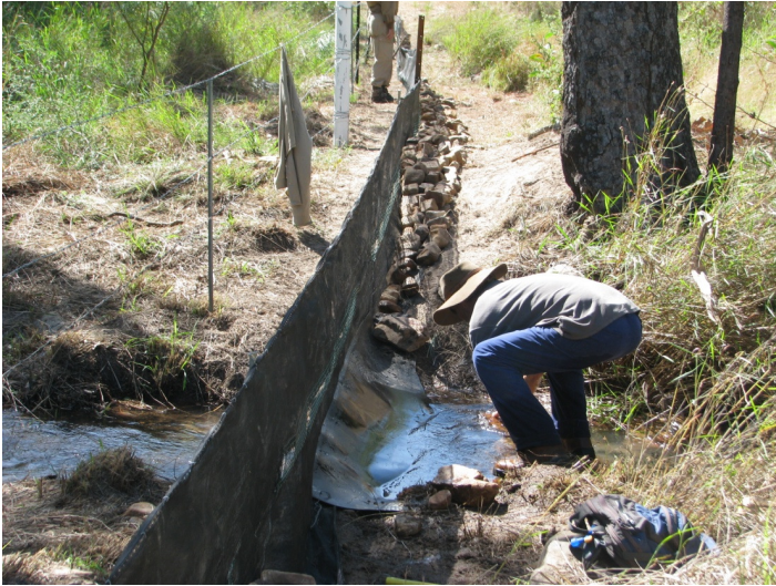
STTF volunteer attaches PVC pond liner material across one of the permanent water crossings.
