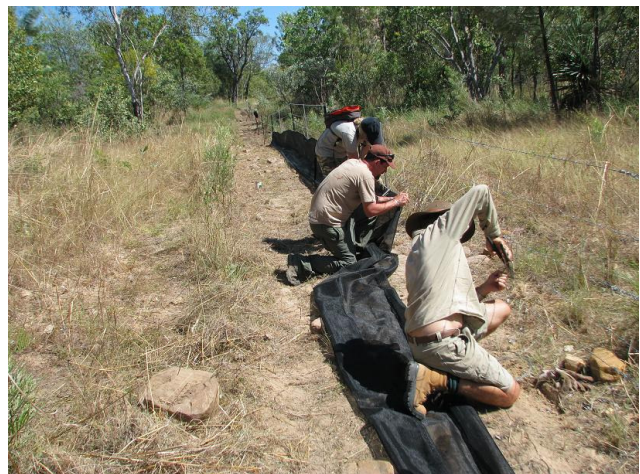
Shade cloth is attached to the existing cattle fence to block the toad's movement into Emma Gorge.
