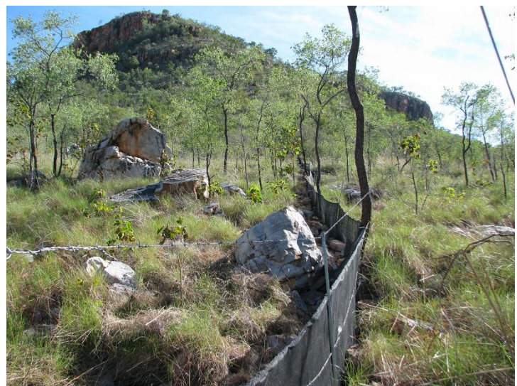
The fence was extended 300m up the rocky escarpment either side by attaching fencing wire to trees.
