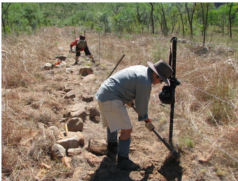
Construction of the fence begins. One of the first steps was to remove any large rocks along the base of the fence to create a flat surface.
