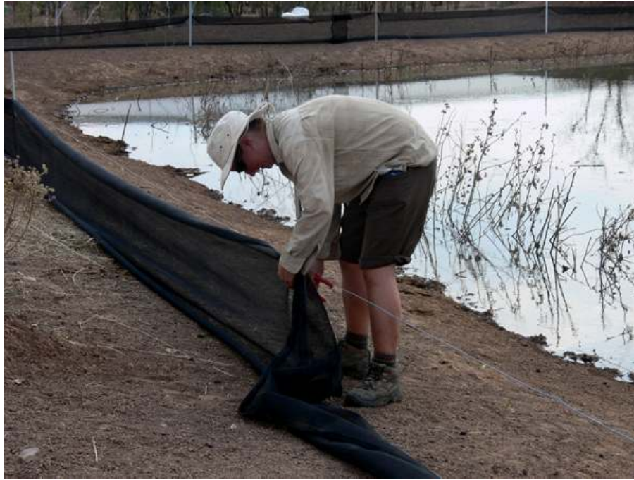
Picture: Volunteer Fiona erecting the fence at Auvergne Station NT- Note top and bottom wires, the overall height of just 50cm, and lack of vegetation inside the fence.
