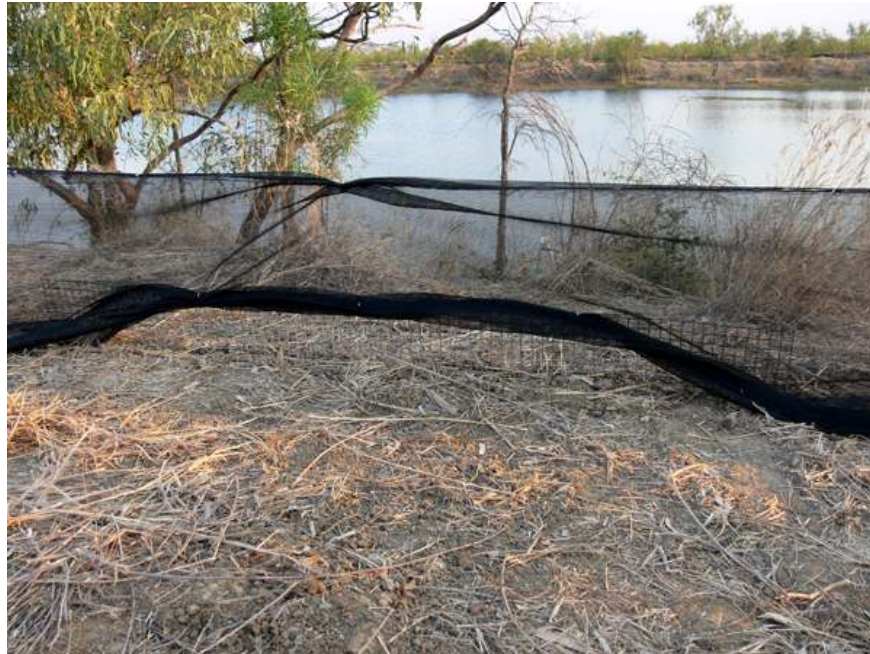
Picture: Native frog gate, made from 25mm square mesh installed in the fence allows native frogs to easily pass through the exclusion fence.
